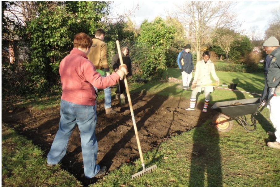
Constructing the foundations to the greenhouse
